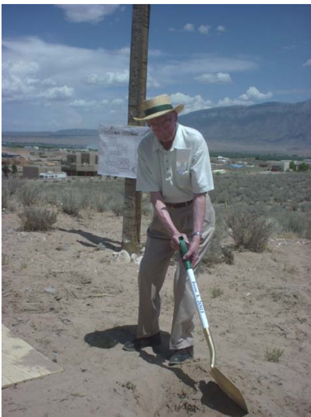
Founding Member Willard Prekker digs the first hole for the new church.
